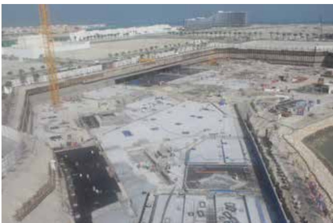
Concreting of raft slab foundation complete
