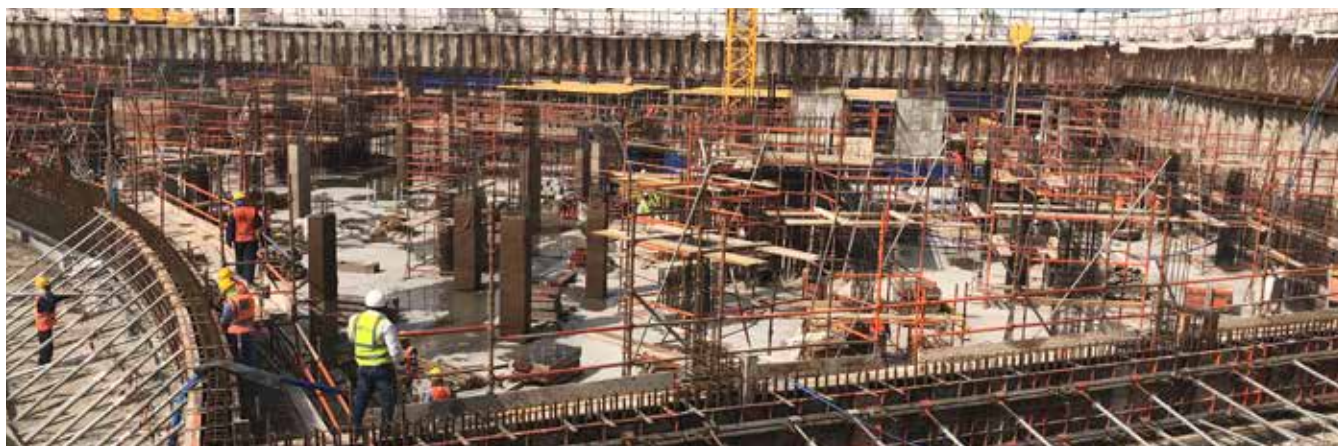
Concreting of upper retail columns
