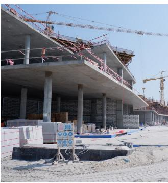
Column Shuttering, Reinforcement and Concreting of initial Amenity level residential block A floor in progress (15% complete)
